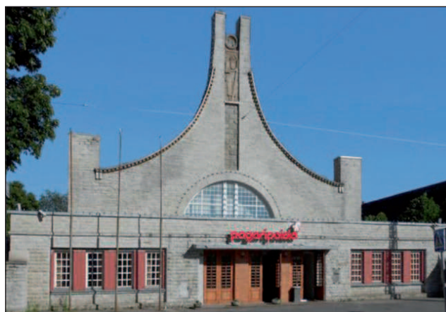
7. Klub robotniczy w Tallinie (proj. Armas Lindgren, Herman Gesellius i Eliel Saarinen). Fot. Jacques Lasserre 7. The workers' club in Tallinn (designed by Armas Lindgren, Herman Gesellius i Eliel Saarinen). Photo by Jacques Lasserre
