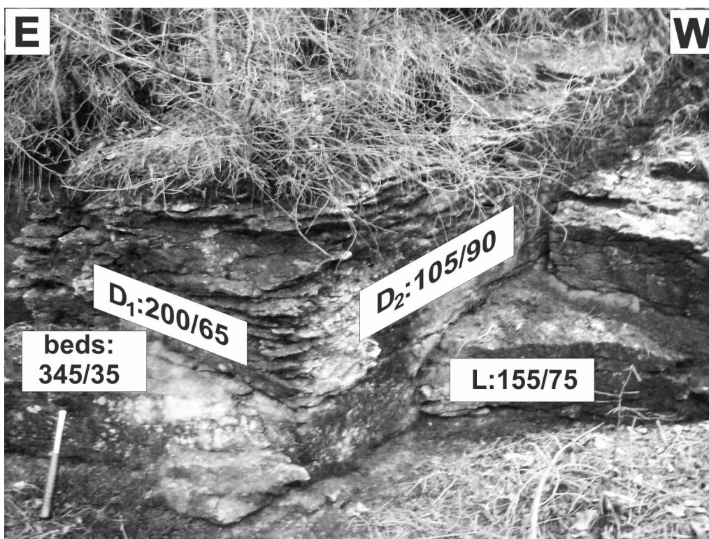
Text-fig. 5. Fractures in the nummulitic Eocene deposits. Exposure on the eastern slope of the Mała Łąka Valley. Fracture sets L, D 1 and D 2 are visible
