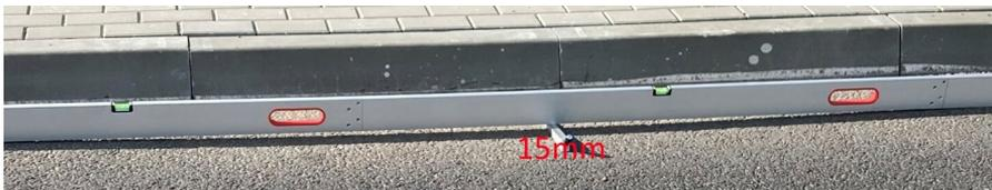
Fig. 1. The view of pavement settlements between column heads
