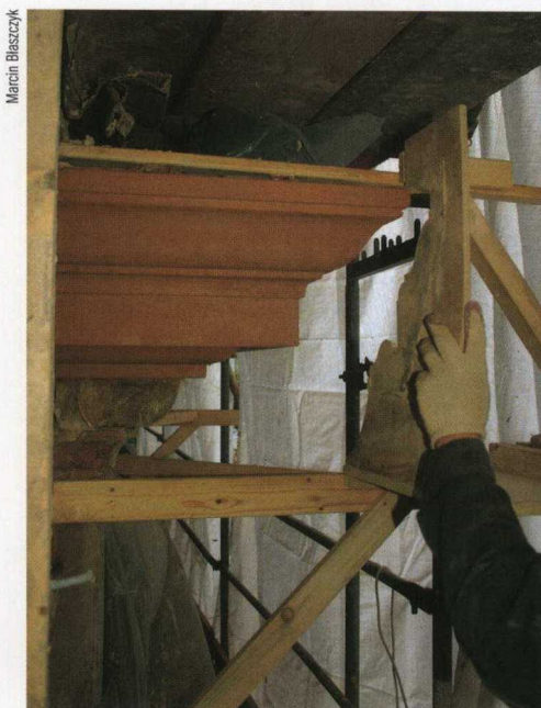
The missing part of this cornice is reconstructed by applying Roman cement mortar and repeatedly passing over a wooden profile
