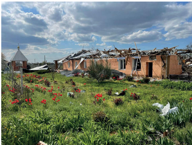
Ill. 5. A destroyed village church in the Mykolaiv Oblast. Photo by S. Belinskyi.
