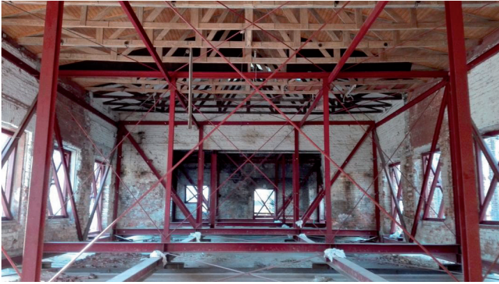
Fig. 7. View of internal strengthening structure of building No. 15
