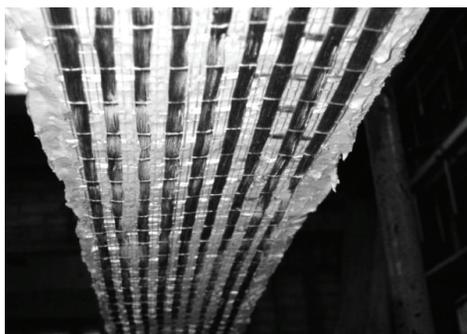
Fig. 5. Ruredil X Mesh Gold after fitting
