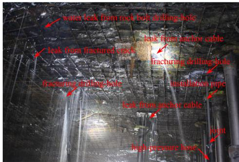
Fig. 12. Conditions surrounding the drilling-hole during hydraulic fracturing
