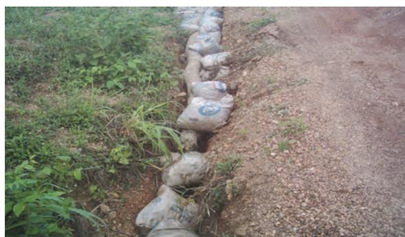
Photo 5. Packs of sand bags as erosion control measures in the study area (phot. O.A. Lawal-Adebowale)
