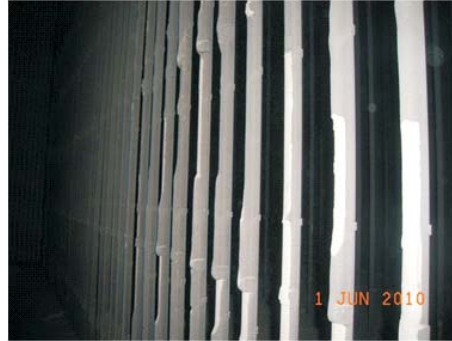
Figure 17. Heating surface of cross channel, the second string.
