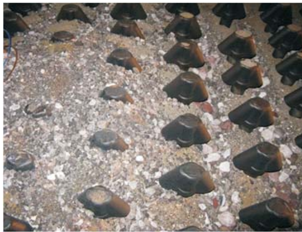
Figure 18. The bottom nozzle CFB boiler, the residual material.
