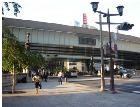
Fig. 4. Elevated expressway above the Nihonbashi Bridge
