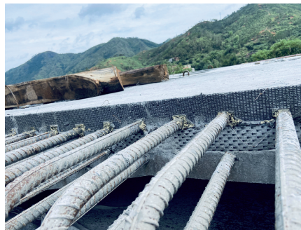
Fig. 11. UHPC overlaid concrete slab of prototype bridge
