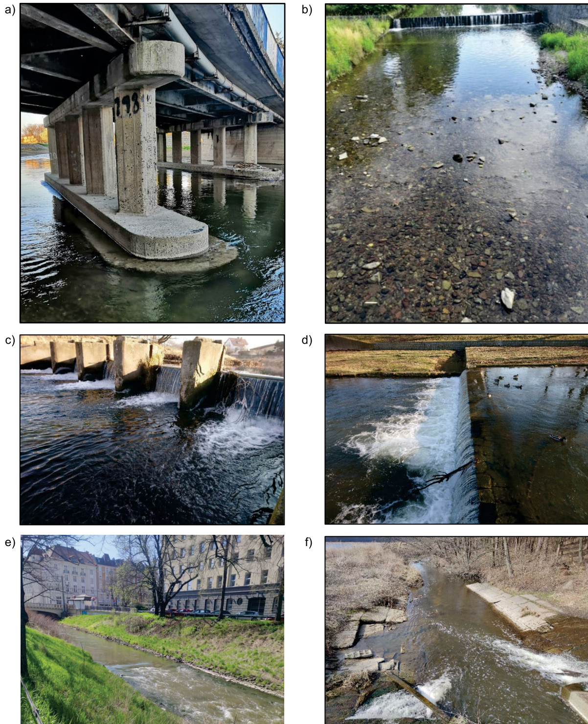
Photo 1. River valley morphological elements included in the River Habitat Survey method: a) bridge piers (the Bystrzyca River), b) visible bottom granulation (the Bystrzyca River), c) concrete weir (the Piława River), d) hydraulic jump visible downstream the stone weir (the Bystrzyca River), e) transition from smooth to turbulent forms of water movement (the Kłodnica River), f) devastated bed and riparian concrete reinforcement (the Czarna River) (phot.: M. Kiraga)
