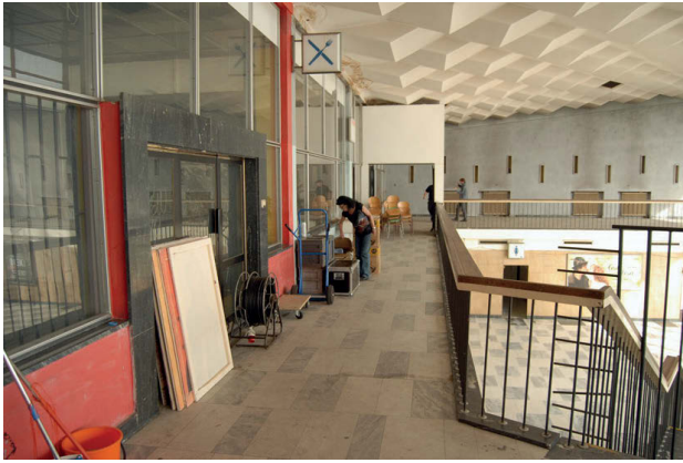
III. 6. Cleaning the gallery before the theatre performance (2012). Source: archive of the Důl architektury association.
