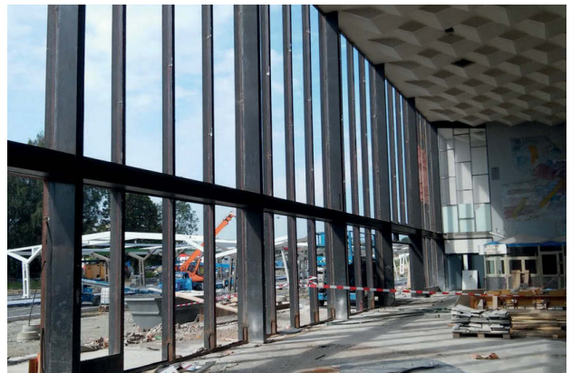
III. 11. Remodeling — without glass facade from the interior (2020). Source: archive of the Důl architektury association.
