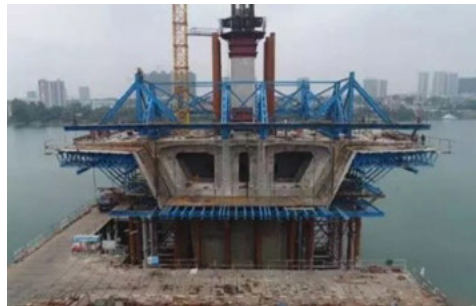
Fig. 1. Bridge with inclined webs box girder
