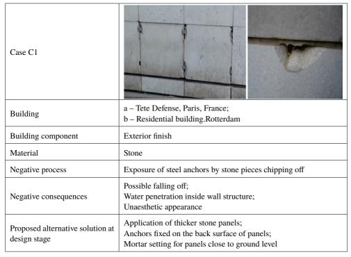
Fig. 7. Damaged stone panels and exposed steel anchors (a – Tete Defense. Paris; b – Residential building, Rotterdam
