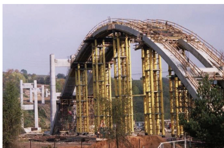
Fig. 6. Concrete arches of Milowka Viaduct a) general view; b) and c) steel scaffolding and timber formwork of arches
