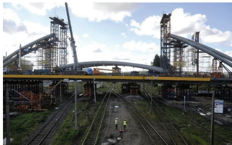
Fig. 12. Viaduct along Slowackiego Street in Gdansk a) general view; b) and c) steel temporary supports
