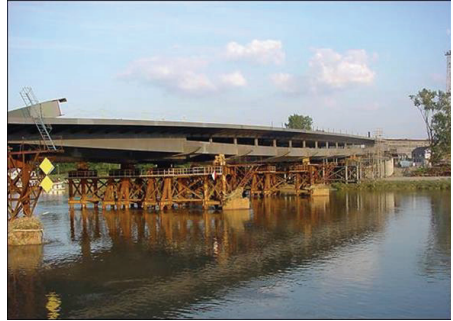
Fig. 18. Kotlarski steel arch bridge over the Vistula River in Cracow a) general view; b) construction of the deck c) erection of arches on steel temporary supports placed on the deck
