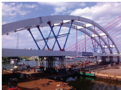
Fig. 30. Steel arch bridge over the Dead Vistula River in Gdansk a) arch divided on three segments; b) superstructure placed on the pontoon; c and d) Transportation of the superstructure on the barge
