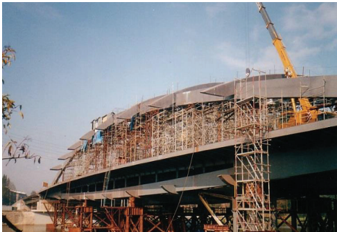
Fig. 18. Kotlarski steel arch bridge over the Vistula River in Cracow a) general view; b) construction of the deck c) erection of arches on steel temporary supports placed on the deck
