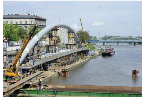
Fig. 21. Bernatka steel arch footbridge over the Vistula River in Cracow a) general view; b) construction of the structure on the riverbank c) floating of the bridge
