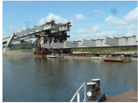
Fig. 15. Steel arch bridge over the Vistula River in Pulawy a) general view; b) placement of the deck c) steel temporary supports for erection of arches
