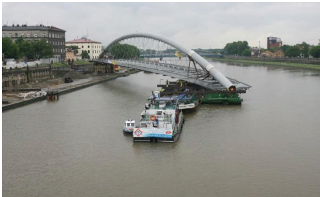
Fig. 21. Bernatka steel arch footbridge over the Vistula River in Cracow a) general view; b) construction of the structure on the riverbank c) floating of the bridge
