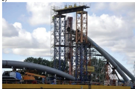
Fig. 12. Viaduct along Slowackiego Street in Gdansk a) general view; b) and c) steel temporary supports
