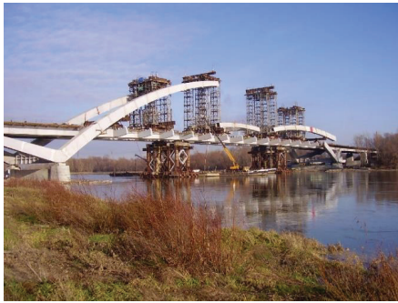
Fig. 15. Steel arch bridge over the Vistula River in Pulawy a) general view; b) placement of the deck c) steel temporary supports for erection of arches
