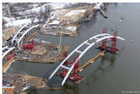
Fig. 27. Steel arch bridge over the Vistula River in Torun a) general view; b) Transportation of the part of the arch on the barge c) fixing of the arch into concrete piers
