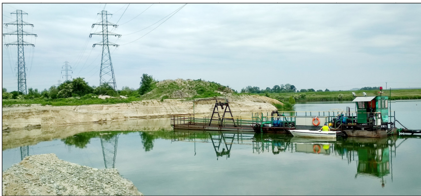
Fig. 2. The “Döpke” dredging machine near the high voltage electric lines
